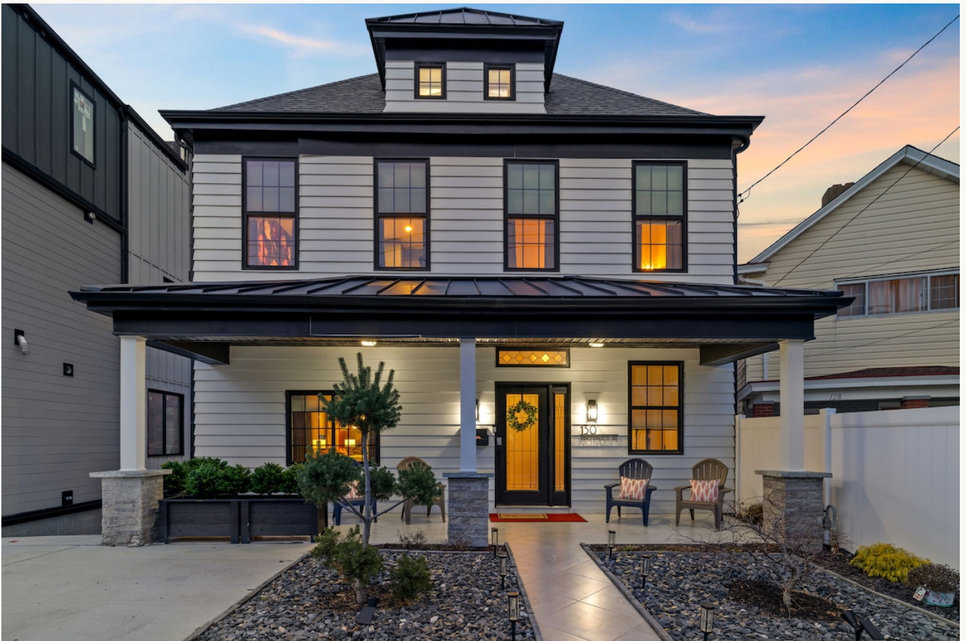
130 Prospect Street / The completed exterior.
